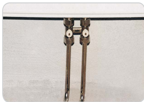
Radiator connection via radiator elbows
