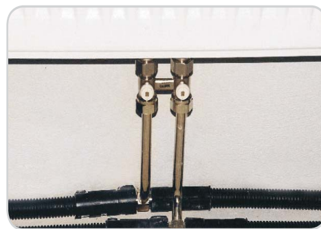
Radiator connection via radiator T-pieces
